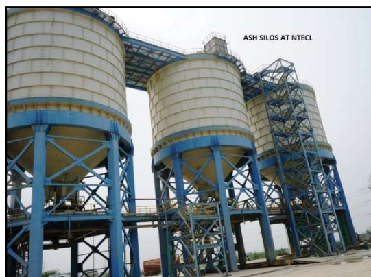
Fig 5: 3 No of Dry ash silos at NTECL
