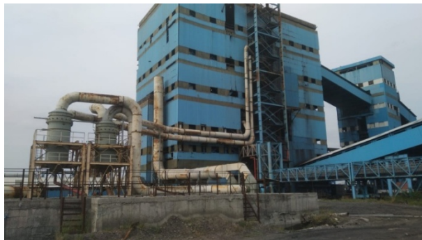
Fig 8: Dust extraction sytem at Coal crusher house
